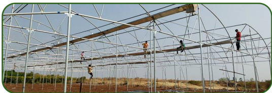
Greenhouse & Nethouse Structure
